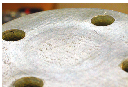
Figure 7. Sinking of gasketing material into surface of FRP flange.
