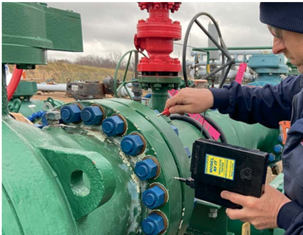
Testing of Flange Insulation Kit
