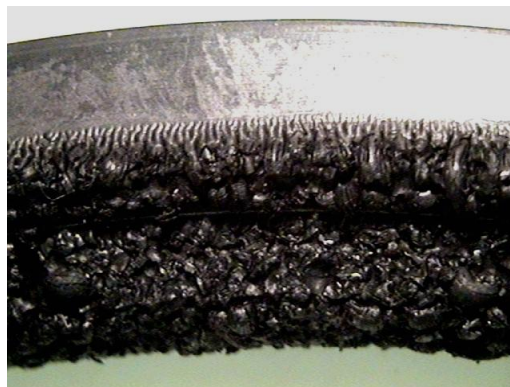
Figure 32 Blistering/ bubbling damage on exposed surface
