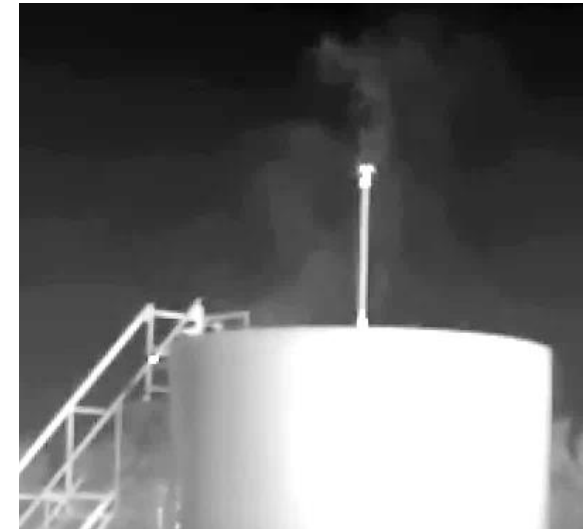
Intentional venting from storage tank
