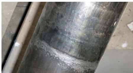
Typical pitting corrosion of a valve stem.
